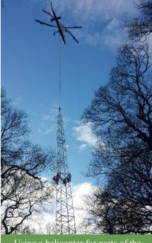
Using a helicopter for parts of the build protected the woodland soil (see "Every breath", above.
